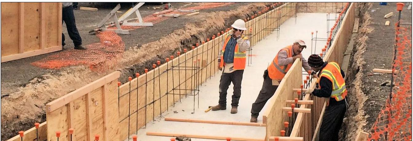
Construction of a bioretention basin at Ramsey Park, parking lot to collect and treat stormwater runoff
